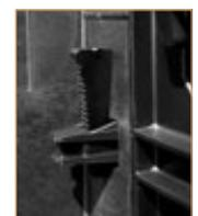
Supporting braces at 1 m intervals join the panels together and strengthen the structure.
